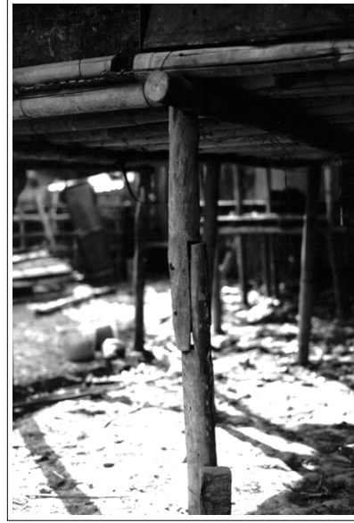
Post with half-lap joint
