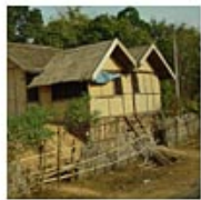
Fig. 12. Double-roofed Lao Loum type.
