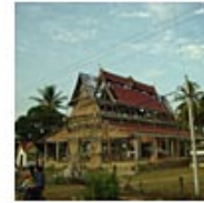
Fig. 27. Temple in building process.
