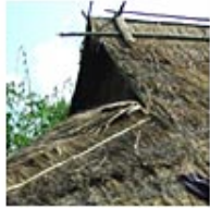
Fig. 32. ...Roof in the house.
